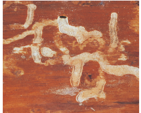
Flatheaded borer tunnel
